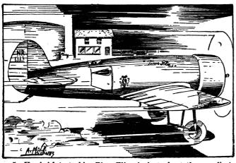
5—Hawks' latest ship, *Time Flies*, is just about the speediest single engined experimental ship in the world. The ultimate in streamlining and powered with a double row Wasp engine which will develop 1,150 h.p. at sea level, it has an estimated top speed of 375 m.p.h. Upon completion of preliminary tests, Hawks expects to continue his record smashing career.
